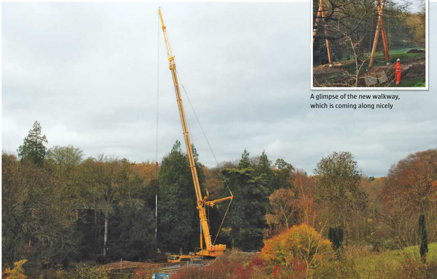
Cranes at work on the Treetop Walkway
